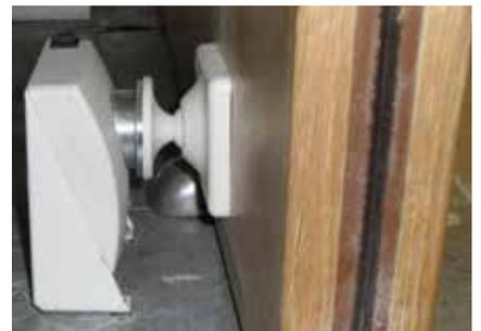
Magnetic door stop. Fire doors on magnetic hold open devices linked to the fire alarm system provide good access and will help to meet the requirements of the DDA.
