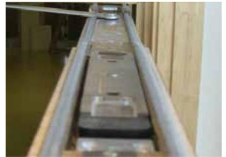
Incompatible security hardware can have a detrimental effect on a fire door.
